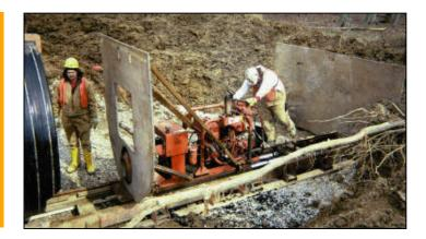
Weholite to be securely grouted without filling the new pipe with water. Even with the old CSP culvert continuing to deteriorate, the 72" Weholite is designed to fully support the Interstate traffic load.
